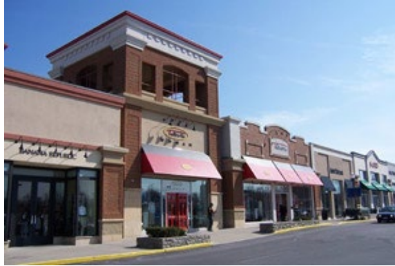
Figure 1228-D: The above image illustrates a building that contains pilasters, cornices, and a series of façade setbacks (recesses) to visually break up the appearance of the large facade.
