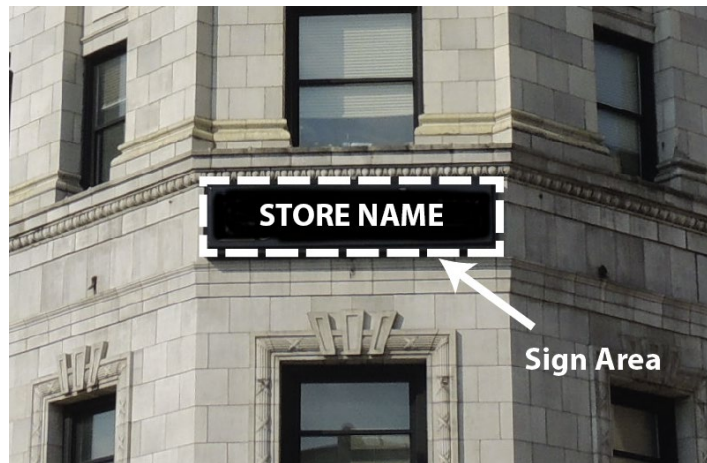
Figure 1236-B: Illustration of computing the sign area for wall signs with a background panel or cabinet.
