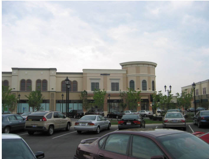
Figure 1228-F: Roofline changes shall be aligned with corresponding wall offsets and/or material or color changes.
