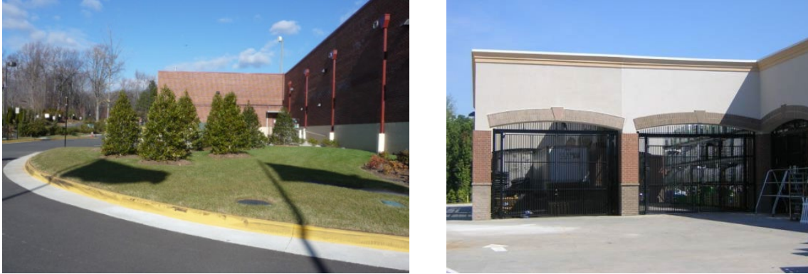
Figure 1232-A: The above image illustrates a vegetative screen that hides HVAC equipment and a dumpster (left image) and the use of a wall and fencing for screening that is architecturally compatible with the principal building (right image).
