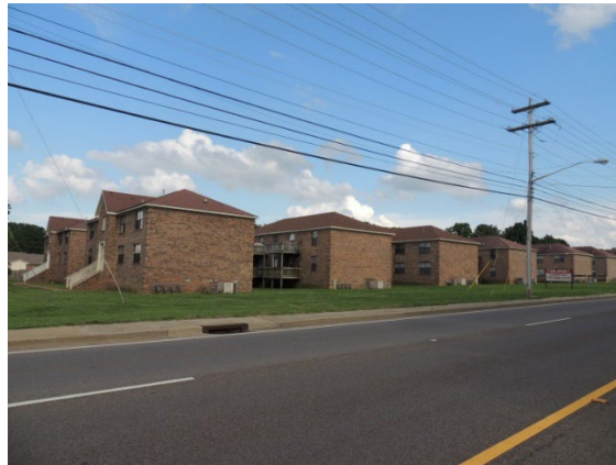
Figure 1228-B: Illustrative example of unacceptable architectural design for multi-family dwellings
