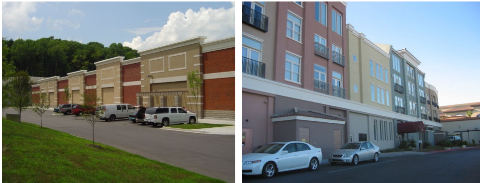
Figure 1228-C: This figure shows two methods of using architectural features to create wall surface relief on wall elevations that are not the primary elevation.
