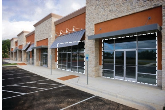
Figure 1236-I: The window area is illustrated within the dashed line area for the two storefronts in the above image. The dashed lines highlight two separate window areas due to the separation by an architectural feature not related to the windows.
