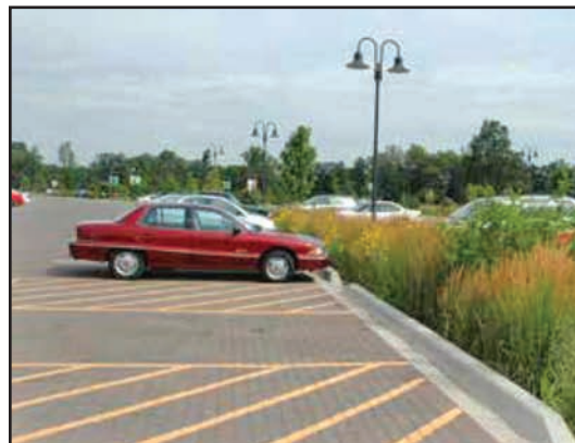
Interlocking concrete pavers with curb inlets to direct rainwater to bioretention area
