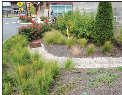
Stormwater infiltration system in parking area
