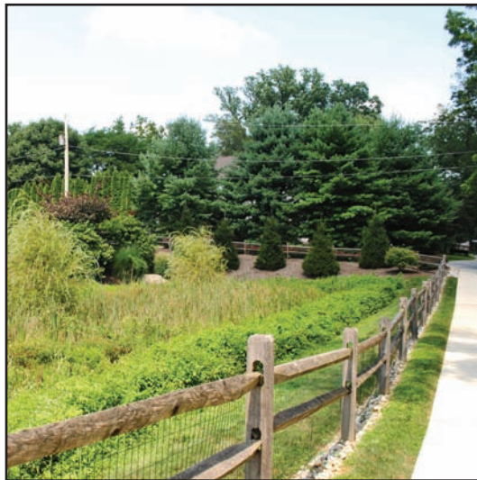
Rain Garden providing Stormwater Management
