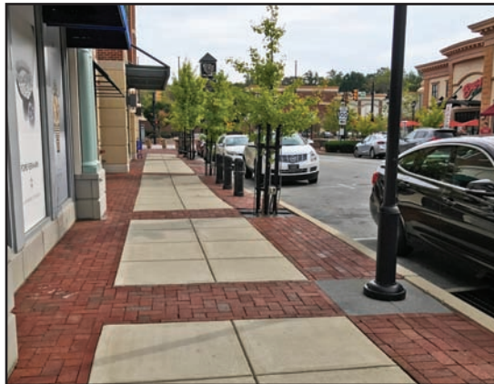
Sidewalks utilizing Unit Pavers
